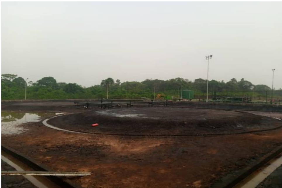
BOLTED TANK DECOMMISSIONING AND ANCILLARY SERVICES
