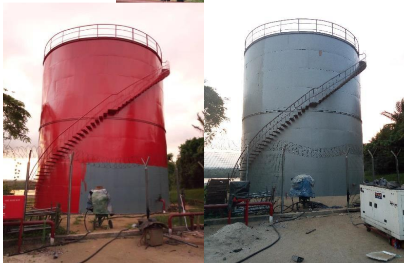
FABRICATION AND INSTALLATION OF VERTICAL TANK
