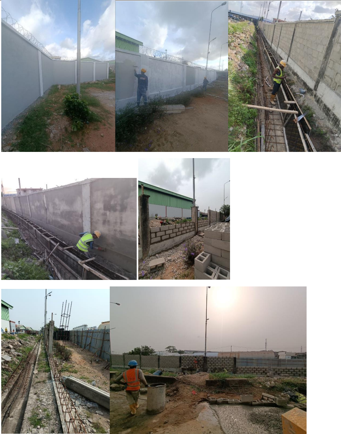
Construction of Perimeter fence at OVH depot
