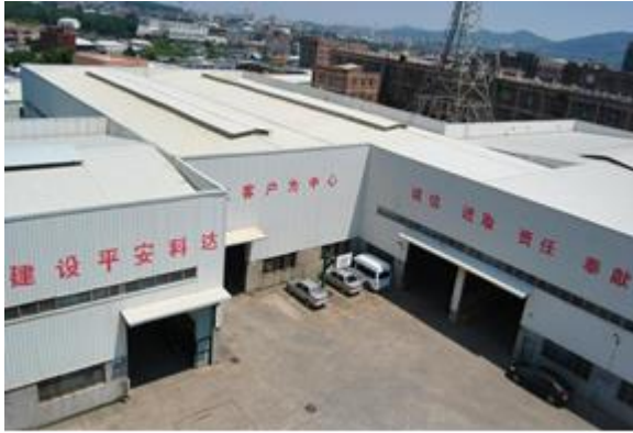
Keda scales manufacture plant overview
